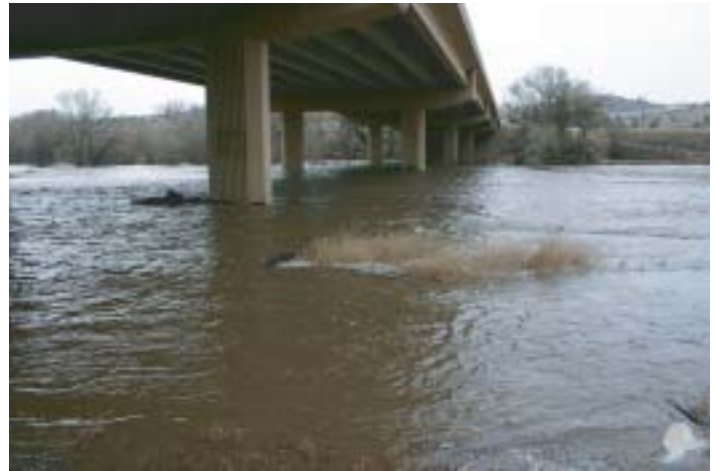
Granite Creek, at the far end of the bridge, is outside its banks. This area below the Prescott Lakes Parkway bridge at Watson Woods Riparian Preserve is typically high & dry!
