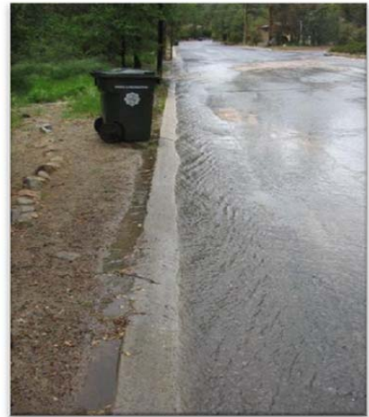
Above: Stormwater flows down Sherwood Drive after a rain storm.
