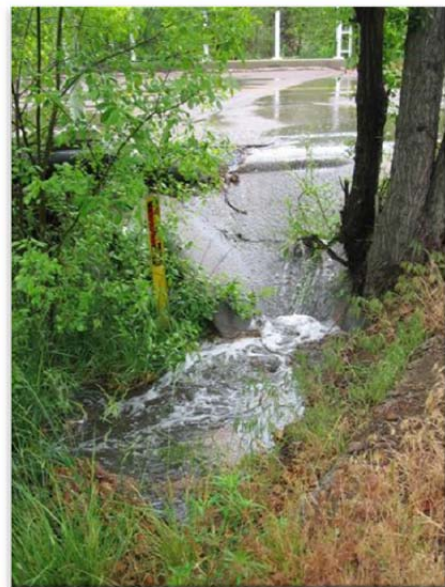
Above: Stormwater from a road drains directly into Butte Creek.
