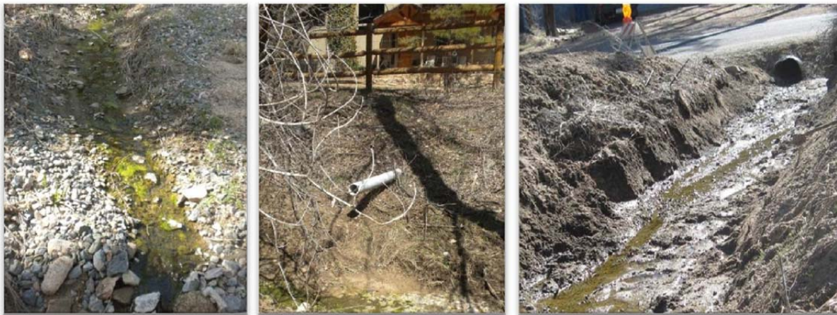
Figure 9: Stormwater Drainage Features
